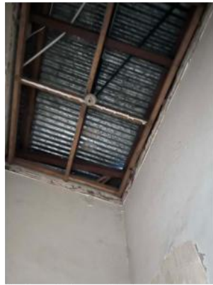
Progress photographs 2.7.2026: Damaged ceilings in the north tower vestibule and old passageway removed. Note the daylight visible at problematic junction of roof with tower wall, and extent of water damage below.
