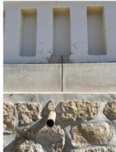
Close-up view of reinstated spout & balustrade 9/6/25
