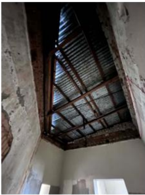
Progress photographs 2.7.2026: Damaged ceilings in the north tower vestibule and old passageway removed. Note the daylight visible at problematic junction of roof with tower wall, and extent of water damage below.
