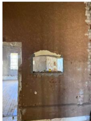
Progress photographs 2.7.2026: Removal of paint and loose plaster in the southern tower vestibule revealing clay, lime and cement plaster beneath, and electrical reticulation.
