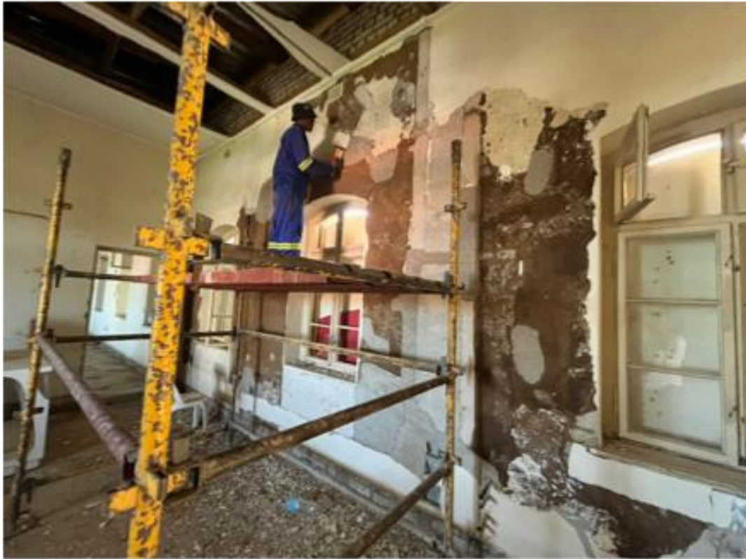
Progress photographs: Views capturing commencement of peeling of paint from the wall surfaces to uncover plaster underneath (25 February 2026).
