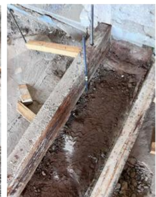
Progress photographs 2.7.2026: Shuttering for floor beams above the old cross-wall foundation walls in the North portion of the West wing is being positioned in preparation for casting.
