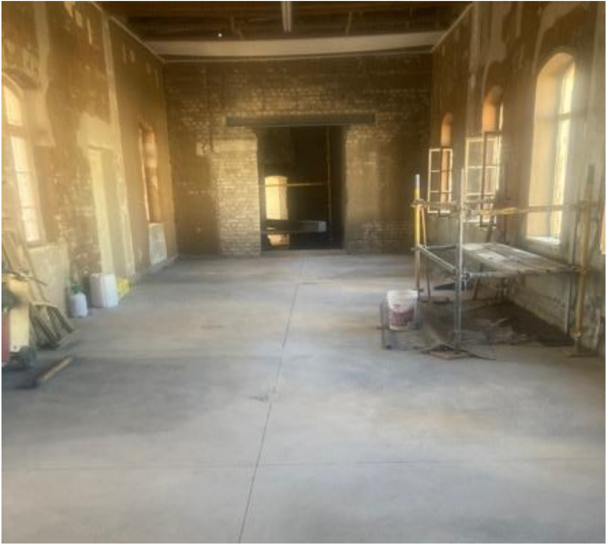
The new floor marks another step towards bringing the West Wing back into use, while the historic walls and windows remain at the heart of the space.
