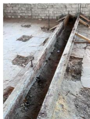
Progress photographs 2.7.2026: Shuttering for floor beams above the old cross-wall foundation walls in the North portion of the West wing is being positioned in preparation for casting.
