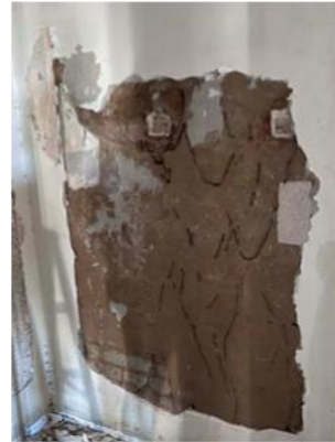
Progress photographs 2.7.2026: Removal of plaster and paint in north tower vestibule underway, exposing original clay plaster. Note the extent of termite activity.
