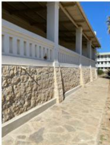
View of completed south plinth & balustrade 19/6/25
