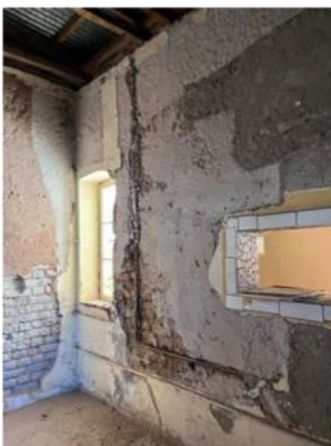
Progress photographs 2.7.2026: Removal of paint and loose plaster in the southern tower vestibule revealing clay, lime and cement plaster beneath, and electrical reticulation.
