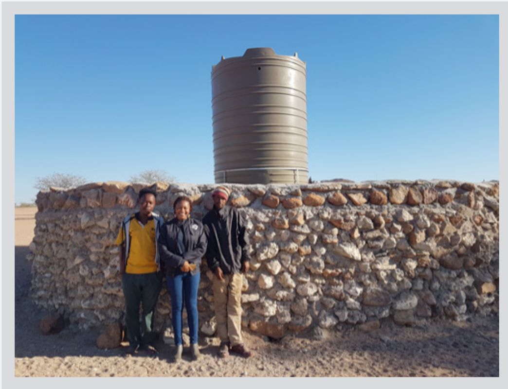
Figure 54 Typical stone wall put up around water infrastructure to prevent elephant damage
