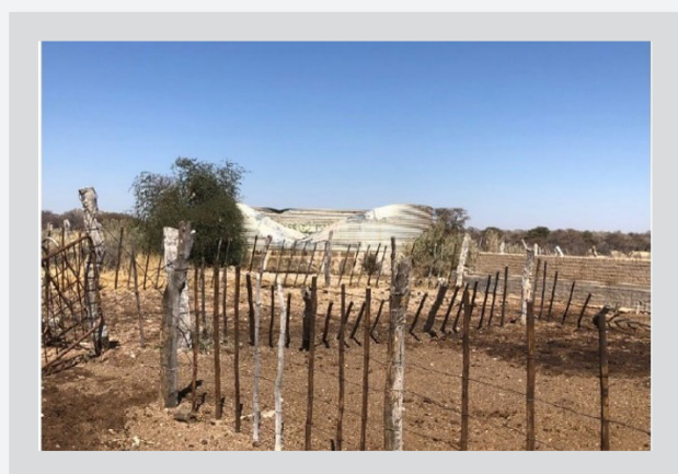
Figure 71 Elephant damage to water and fencing infrastructure on commercial farms near Omatjete (Photos: A. Koch)
