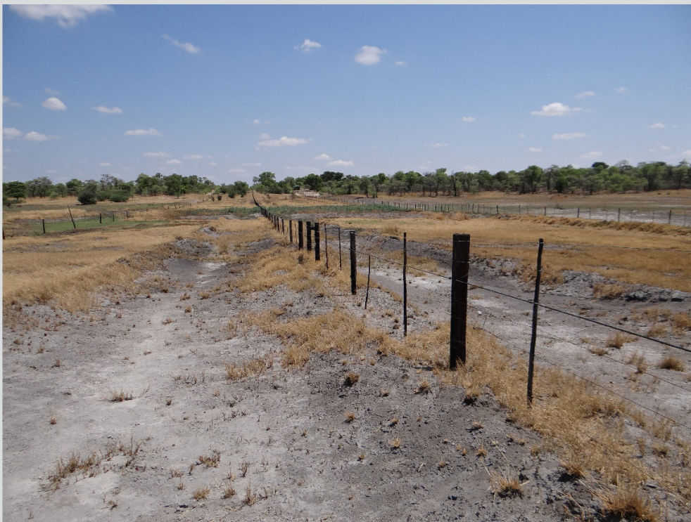
Figure 39 Fences between Khaudum NP (on the left) and western Ngamiland (on the right). The left-most fence is Namibian, the middle and righthand fences are part of the veterinary cordon of Botswana. Note the low height of all the fences and the cable strand in the fence in the middle.
