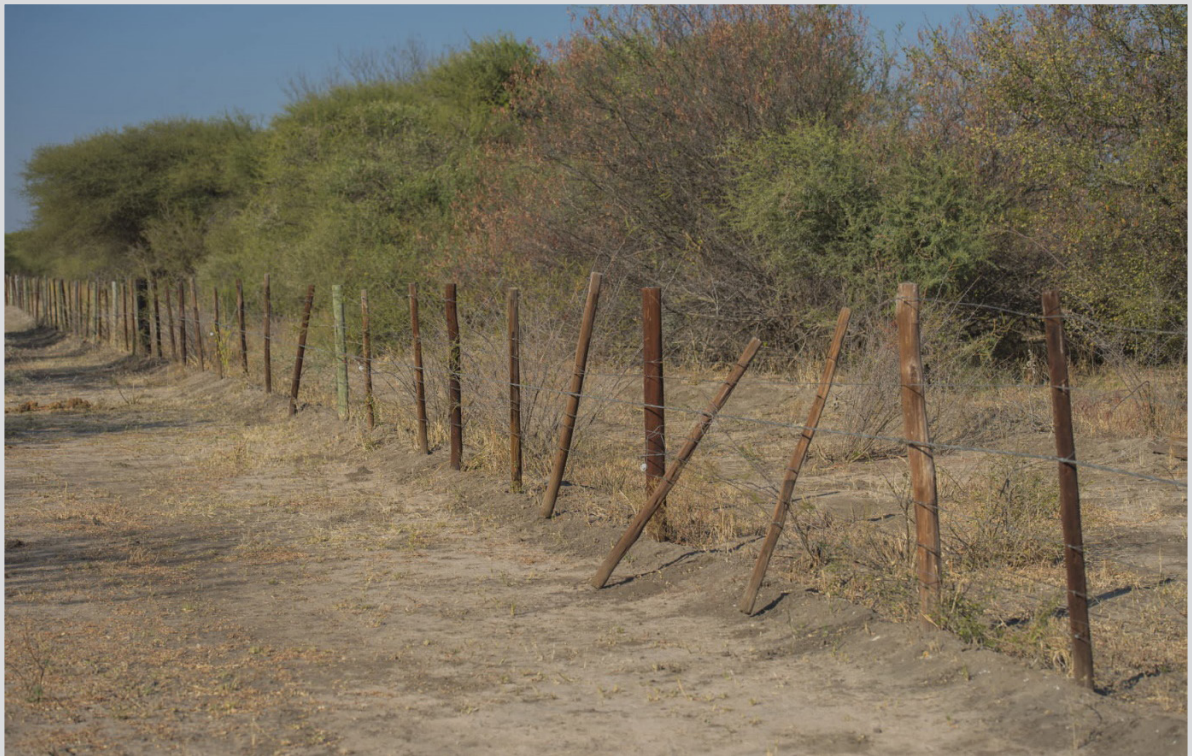
Figure 38 Highly effective fence erected by Botswana on the boundary with Bwabwata NP, consisting of five wire strands reinforced by mesh (in some sections only) and electrified (possibly only in some sections but not maintained). Note that the steel cable is in place of the 4th or 5th wire strand from the bottom, and as shown in the photo largely maintains the integrity of the fence even if larger animals cross it.
